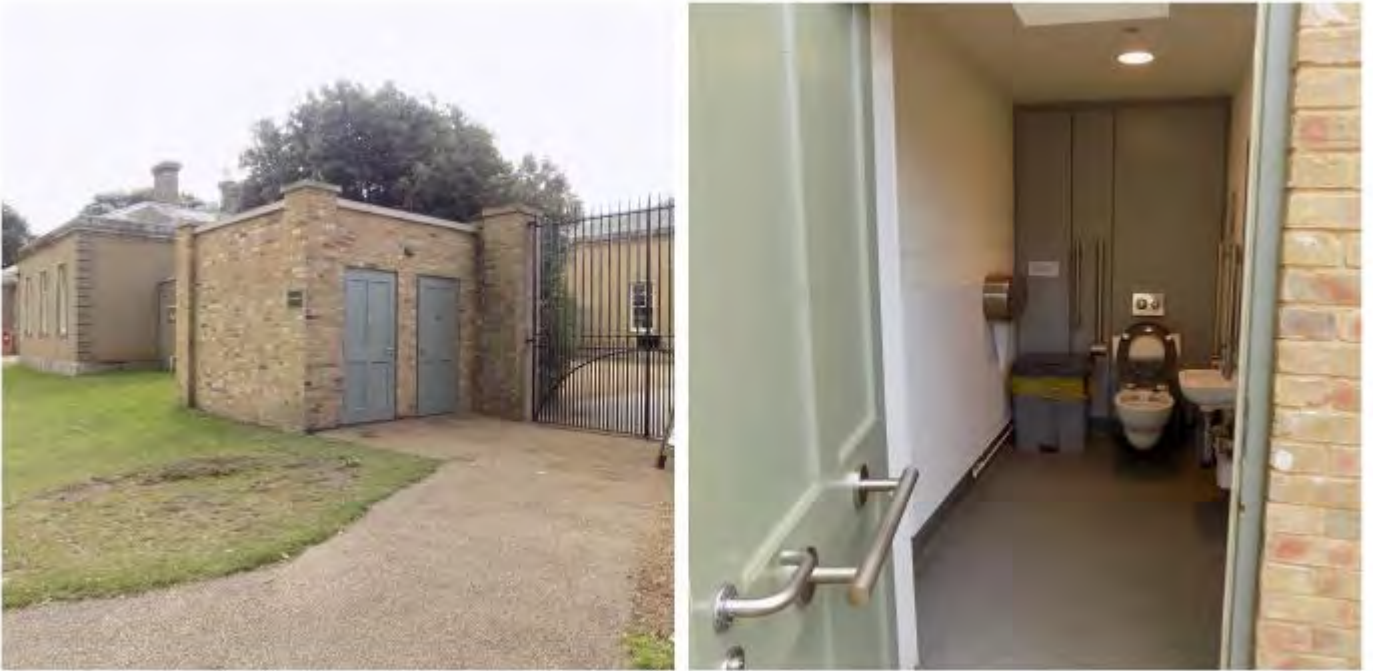
Above: Behind the Visitor Reception there is level access to some toilets, including an accessible toilet. The path is hard surfaced.
